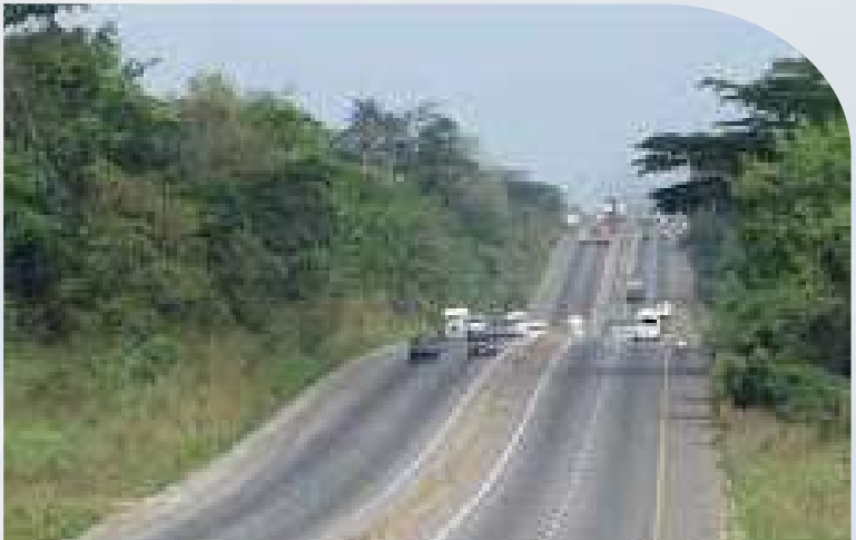
Edo State Ministry of Infrastructure: Road design standards, specifications, and quality assurance for transport systems
