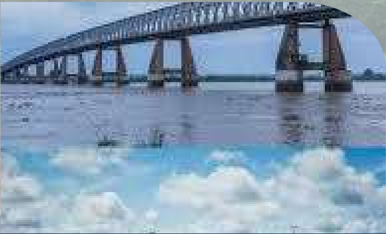
Construction of the 2 nd Niger bridge linking Anambra and Delta states through a concession under the Public Private Partnership (PPP)
