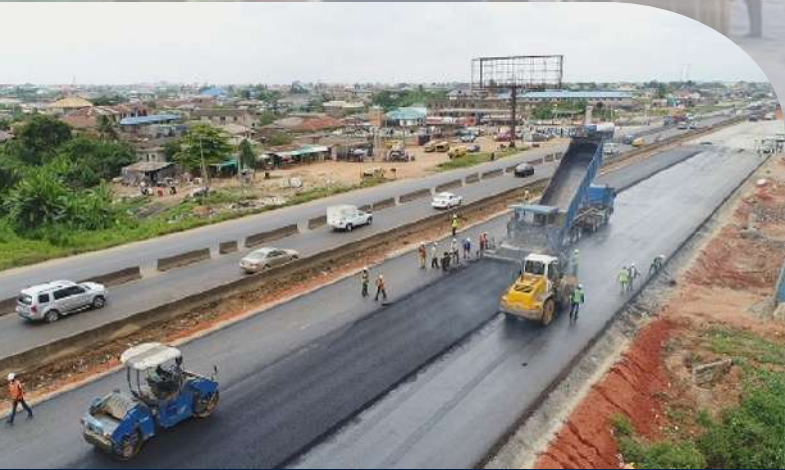
Design and bidding documents for Edo roads using Geo-Nano technology to extend pavement life and reduce costs, funded by Federal and State Government
