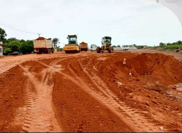
Development of Design, Build, Finance, Operate, and Transfer (DBFOT) of the Benin to Ekpoma Highway in Edo State
