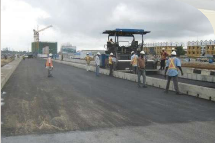
DBFOT Development of FESTAC Phase 2 Internal Roads and Mile Two–Badagry–Airport Bypass
